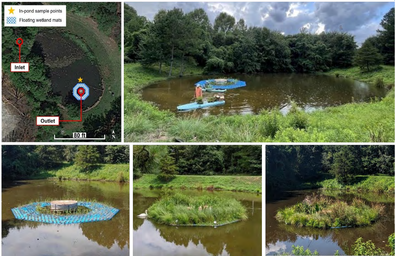
Armory Pond FTWs; top row: aerial imagery depicting FTW design and water quality sampling locations (left) and FTW installation (right); bottom row: FTWs directly following installation (left), approximately 12 months following installation (center), and approximately 24 months following installation (right).
