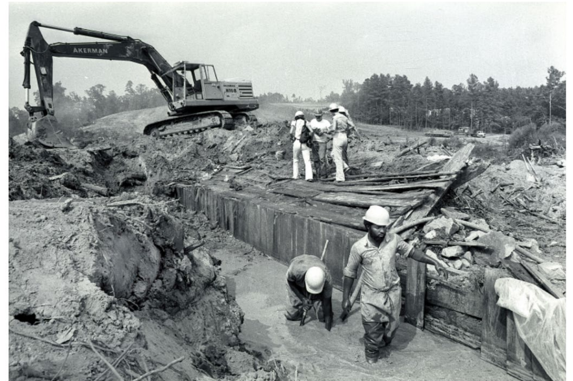
Photograph of workers on an old wooden dam uncovered during construction of Falls Lake Dam in the late-1970s. When this photo was taken, the wooden dam was over 150 years old and covered by silt, mud, and water. Photograph courtesy of the US Army Corps of Engineers.
